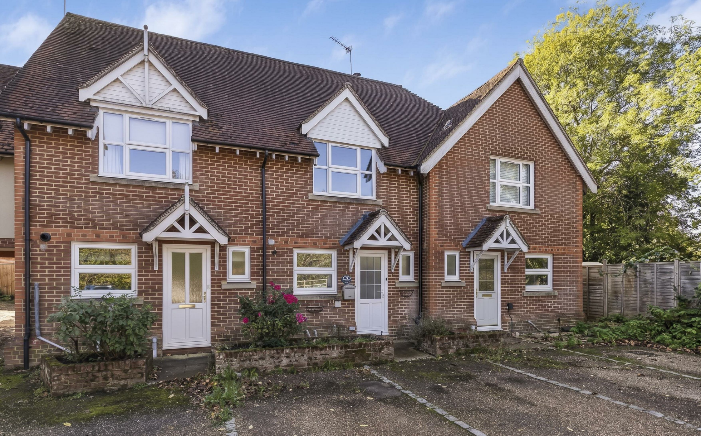
Claywall Cottages, Steeple Bumpstead, CB9 7BZ
